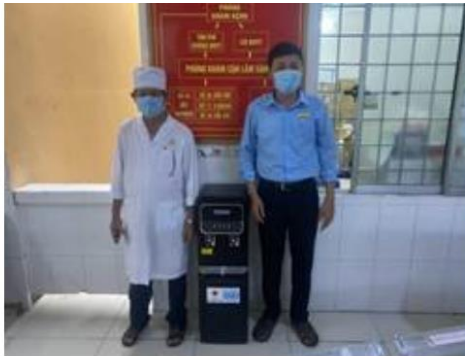
Country: Viet Nam Company: Tromso Co., Ltd. Installation of the water purifier
